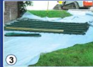
Connect Multiple Stabilizer Grids Using One Of The Following Stapling Methods
