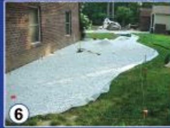
Wash Stones And Allow To Dry (Or Use Gravel-Lok Pebbles). Mix Stones With Gravel-Lok In A Cement Mixer Or Wheelbarrow
