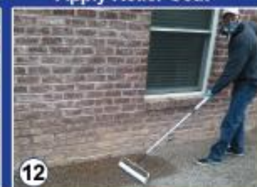
Apply Roller Coat
